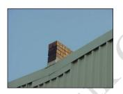
Leaks into the property. Brickwork weathered. Both go to valley gutters which are leaking into the property.
