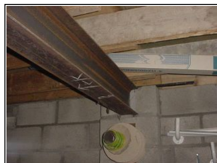
Added RSJ forming support for the first floor timber joists above
