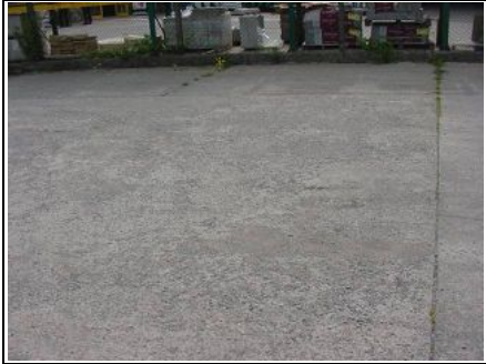
View of car park with a spalling surface
