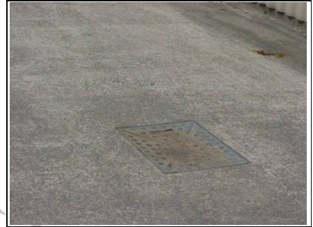
Lightweight manhole cover in car park and has dipped
