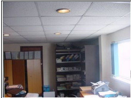
Square ceiling tiles within exposed grid in office area
