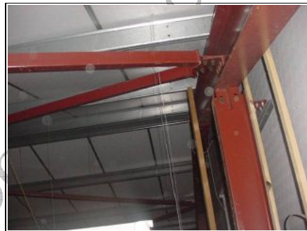
Bolted together wind brace
