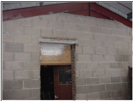
Fire break without the fire door!
