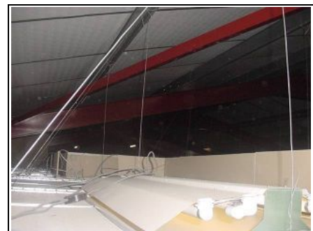
Shows the partitions raised above the suspended ceiling but not to the roof to form a fire break
