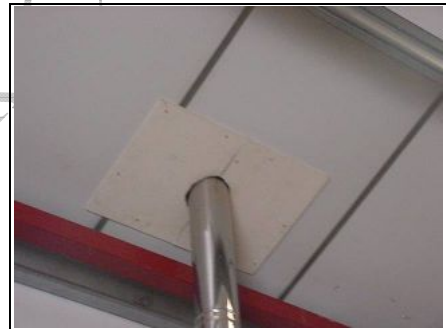
Possible asbestos where flue goes through roof
