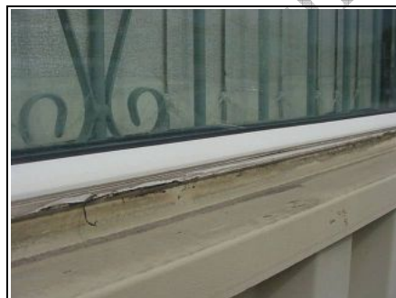
Plastic windows close up. Plastic sill needs re-sealing
