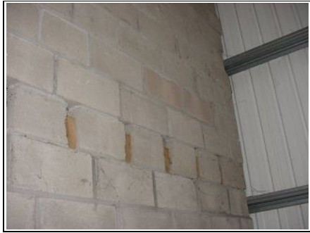
Joists not sitting into blockwork walls properly – DIY Standard
