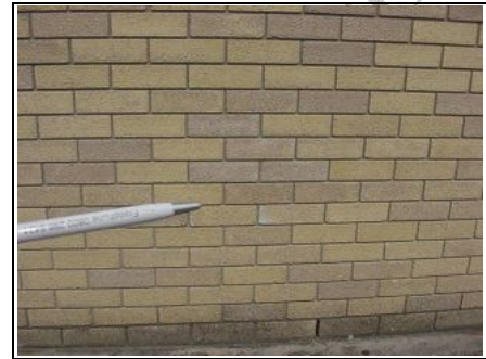
Stretcher bond brickwork
