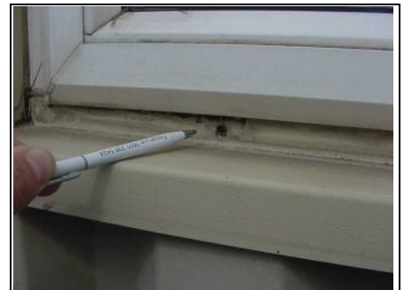
Fixing bolts missing altogether need to be replaced
