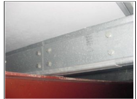
'I' beam supporting purlin which then supports the under cladding.
