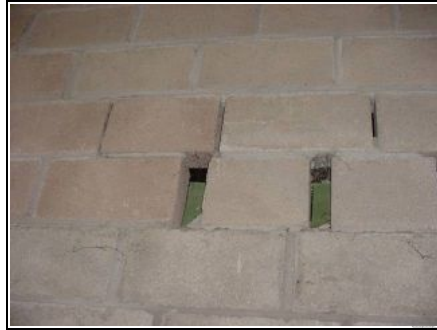
Joist ends not properly supported
