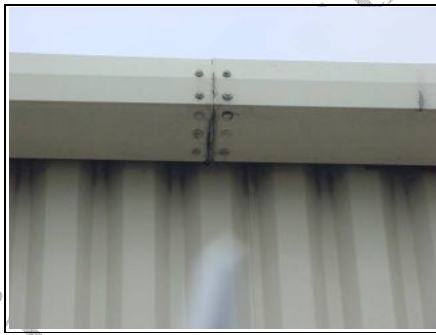
Close up of leaking gutter
