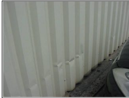
Low level impact damage – very difficult to repair and much better to put a barrier up to stop the cars running into it.
