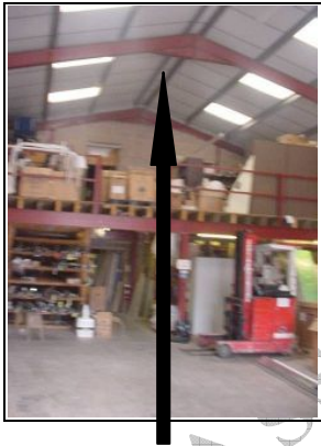
General view of metal portal frame roof
