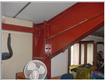
Wall 'I' beam meets roof purlin
