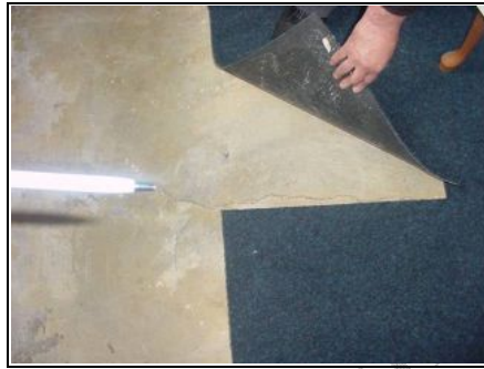
Cracked joints
