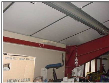
Silver metal purlin gaining support off the portal frame
