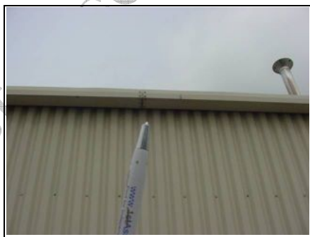
Leaking gutter
