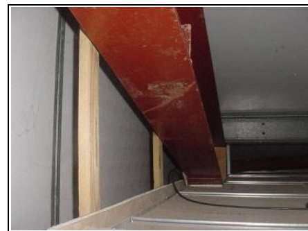
Dry lining in front of wall cladding (front left hand side)
