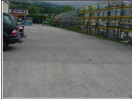
View of car park with a spalling surface
