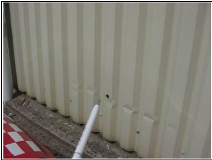
Impact damage caused by cars
