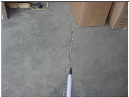
Pen indicates hairline cracking
