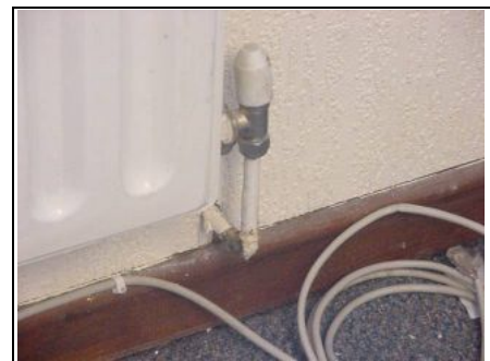
Microbore pipes
