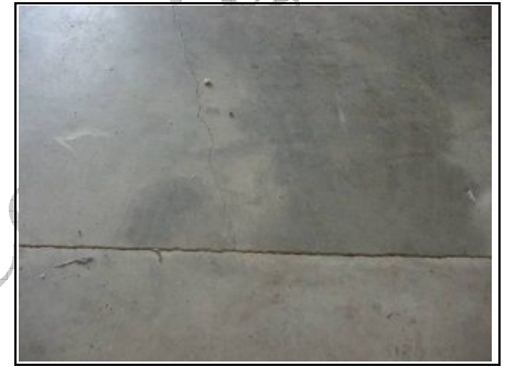
Construction joint
