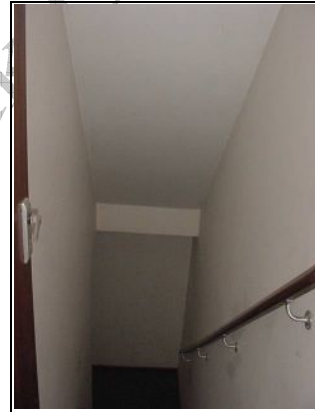
Fire escape plasterboard ceiling
