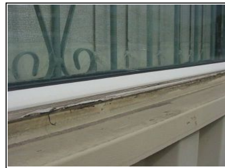
Mastic seals going around the windows would benefit from being repaired.
