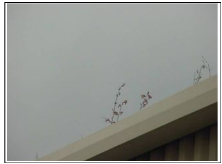
Vegetation growing out of gutter
