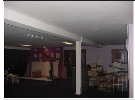
Plasterboard ceiling in show room area, we assume on to a joist and floorboard construction above
