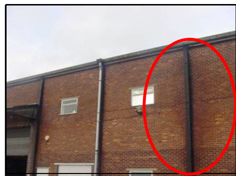
Damp staining to brickwork from leaking gutters
