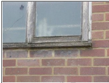
Close up of window in need of repair and redecoration
